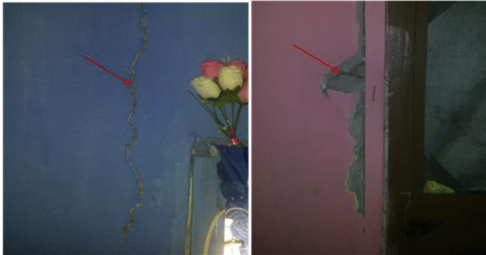
Fig. 3 – Cracks in the walls (bedrooms) of Building Structures at Nkanponase. Residents attribute the cracks to blasting activities by small scale miners.
