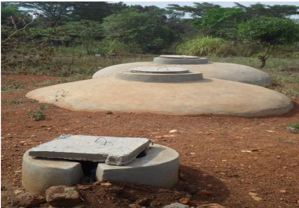
Figure 28: Biolatrline system showing expansion chamber (front view)
