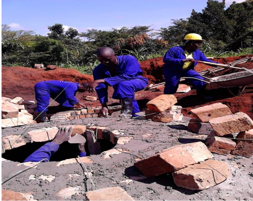
Figure 27: Artisans during Practical construction of the Biogas Digesters
