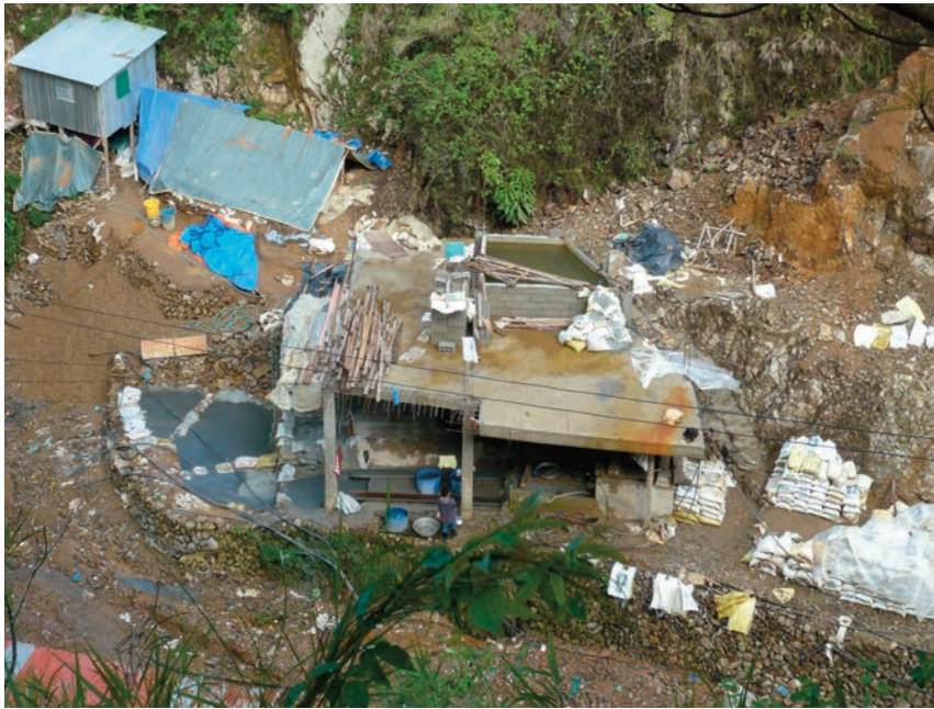
Fig. 6-6. Heap leaching a pile of tailings with cyanide. The plant is sheltered by a blue tarpaulin to reduce evaporation of the cyanide.
